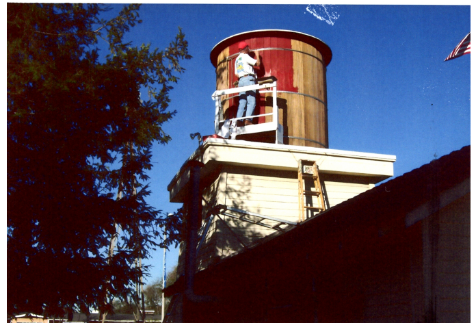
Frank puts the finishing touches on the water tower
